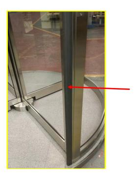
Corner post (Entry point) sensors are heavy duty rubber compression sensors which stop door rotation when compressed by a person or an object. They are active to 48" above floor level.
