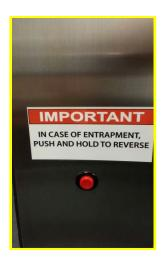
In the extremely rare case where the door does not complete full rotation and stops with a user within the revolving door, there is an Entrapment Release button on the interior center mullion of the door. **PUSH AND HOLD** this button until the door starts to rotate in reverse. The user must exit the door when the door has stopped rotating.
