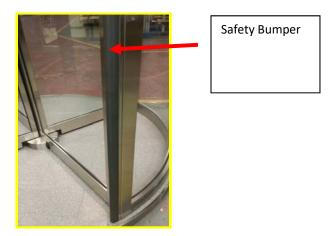
**Step 2** – Enter the revolving door. The presence sensor in the door section ceiling will pick up the user and will start to rotate automatically. **DO NOT PUSH THE DOOR WINGS**. The door wing will rotate 180 degrees allowing the user to pass freely from the non-secure side to the secure side (interior).
